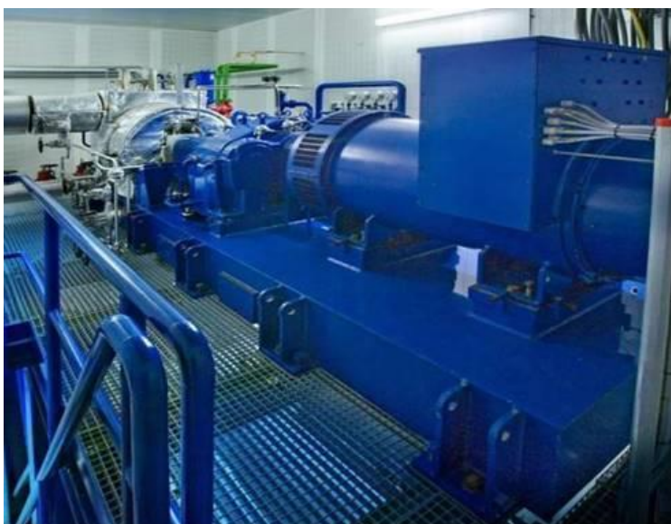
Figure 5.4: Steam turbine
