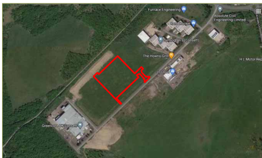
Figure 3.1: Aerial Photograph of the Site
